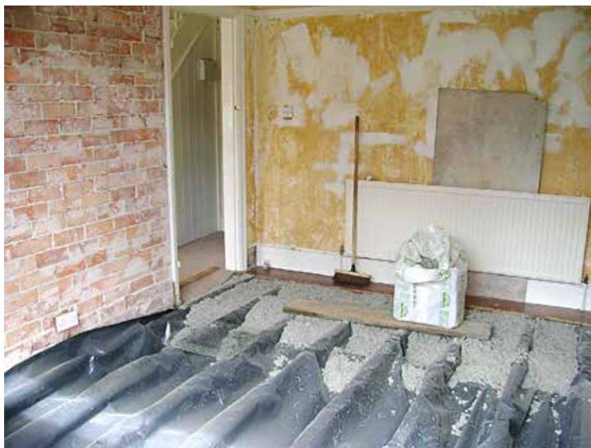
Underfloor insulation going in
