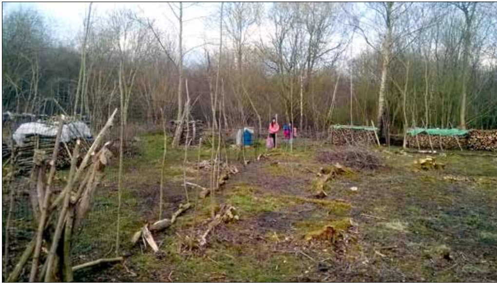
Erecting a deer-proof fence in the wood
